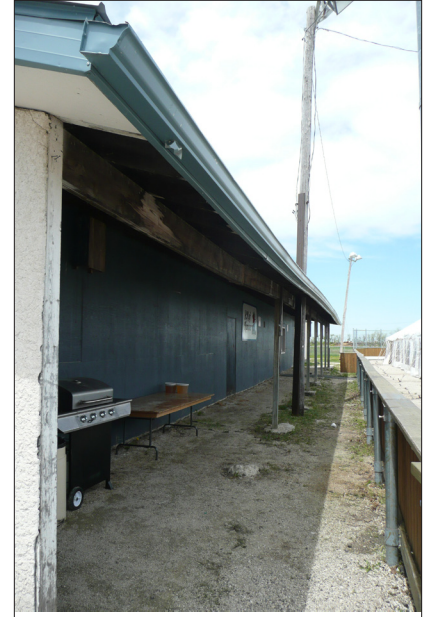
Community Hall Upgrade
